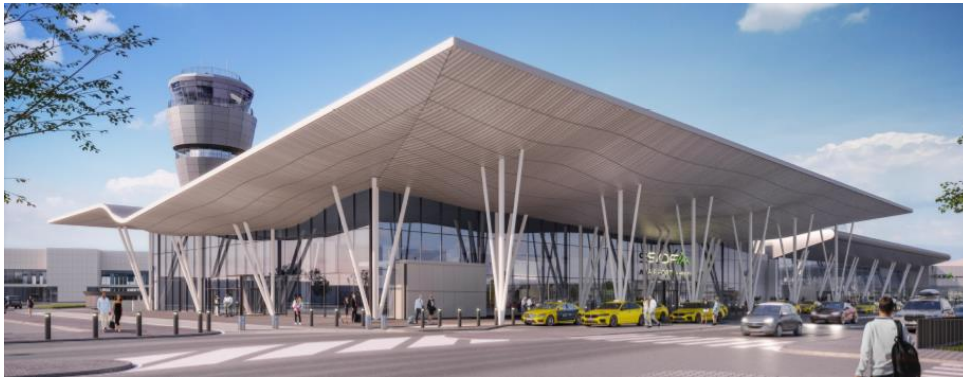
New Terminal T3 – Landside facade Arrival Hall
